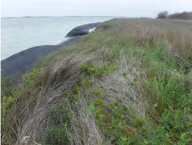
Picture 37: RU010JLM Bearing: East Date: 4/27/2021
