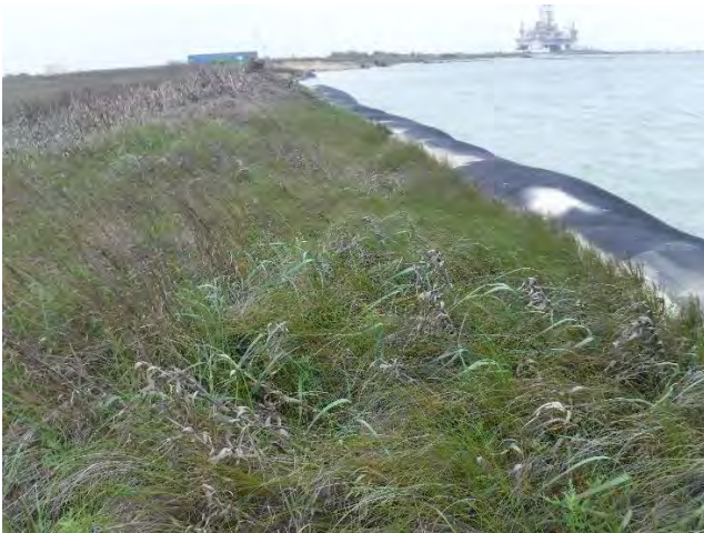
Picture 39: RU010JLM Bearing: West Date: 4/27/2021
