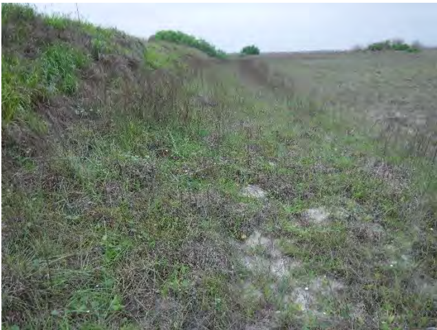
Picture 27: RU006JLM Bearing: Southeast Date: 4/27/2021
