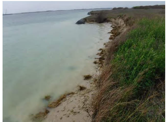
Picture 34: RU009JLM Bearing: East Date: 4/27/2021
