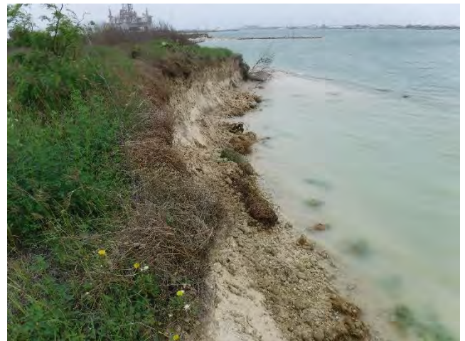
Picture 36: RU009JLM Bearing: West Date: 4/27/2021
